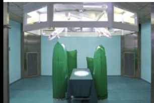
The new laminar air ceiling
